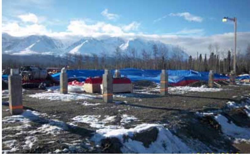
The Dä Kų Cultural Centre construction site this October
